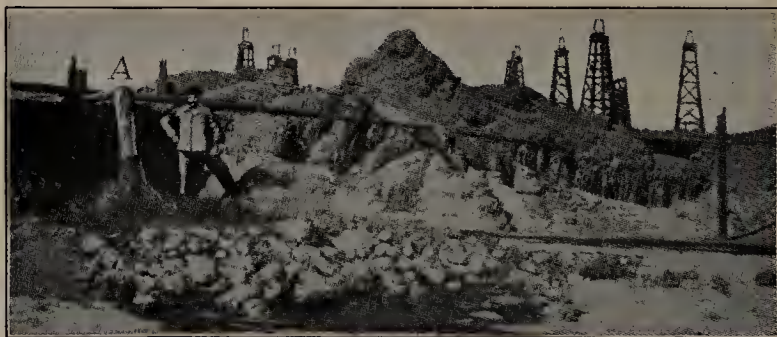
FIG. 91. Forcing liquid sulfur from deep wells in Louisiana by means of compressed air
